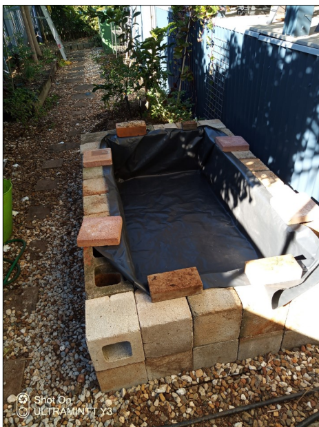
Blocks with plastic liner in place
