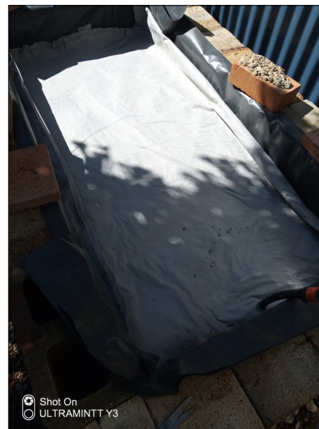
Geotech permeable layer
